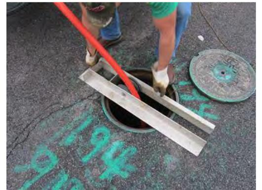
12. Select the proper size debris trap and attach the appropriate number of extension poles needed to place the trap in the manhole channel.
