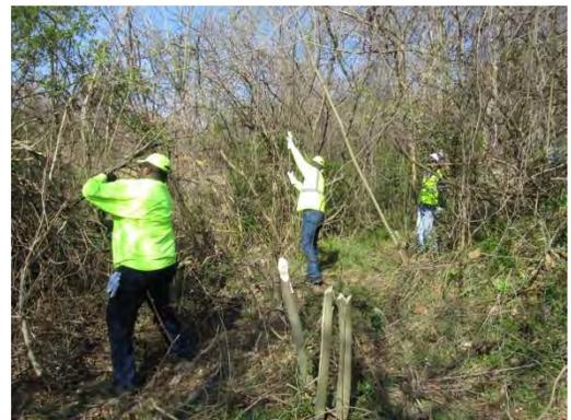
NOTE: Easements are typically cleared in sections: one section is fully cleared, then a path is piloted into the following section. This process is repeated until the entire length of the easement is cleared and all manholes and cleanouts have been located.
