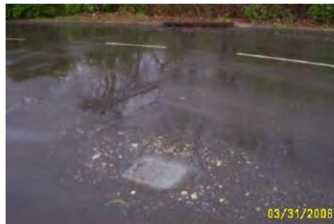
Private Sewer Overflows at strip malls- The inspector needs to make the FSE manager/owner aware of problem, and request that any private plumbing company that cleans the private sewer lines should contact the sewer maintenance personnel to ensure that large amounts of FOG are not pushed into the downstream sewer system and cause another blockage. Also, the Health Dept. should be contacted, which in many cases will result in the closure of the FSE(s).
