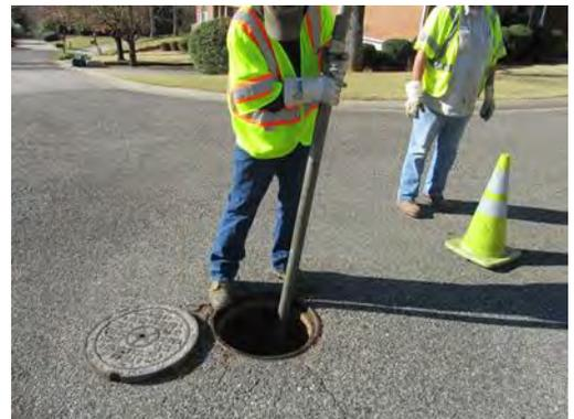
If a larger tool is needed to clean the pipe, remove the rigid pipe set up from the manhole and replace the tool. Repeat the cleaning process.
