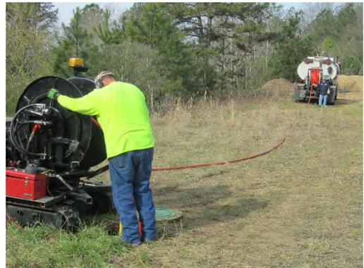
20. Use the trap or a pincher shovel to remove the solids, or consider using the vacuum system to remove the solids.
