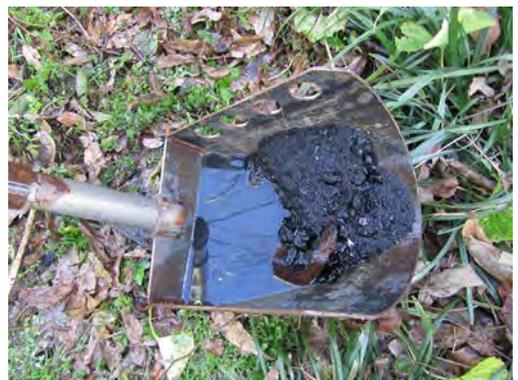
21. Place the material removed from the manhole into burlap bags or 5-gallon buckets.
