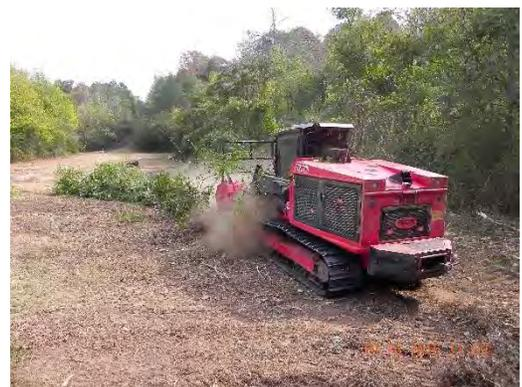
4. Use heavy equipment to cut down brush and small trees to the limits of the easement.
