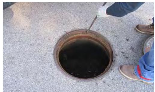
5. Confirm that the manhole depth, pipe diameter, and material match the manhole description on the work order.
