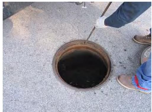
If the guide pipe is not long enough to reach the manhole invert, thread more sections of pipe onto the guide pipe.
