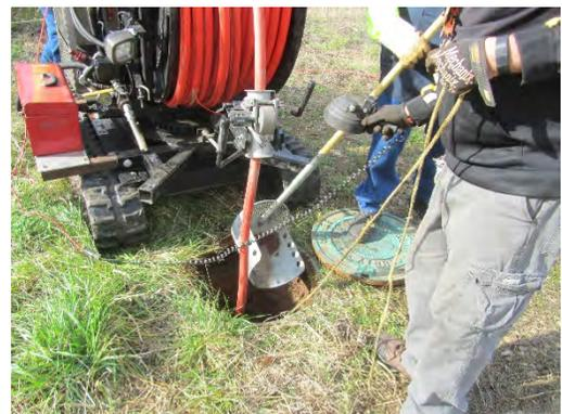
13. After checking the headset radio is functional, or by using hand signals, coordinate water delivery to the easement machine to start cleaning operation.
