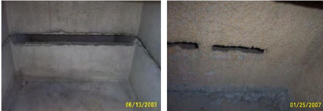
Slit style baffle walls, are not as efficient as the single hole baffle wall design
