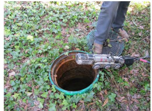
11. Measure the depth of the manhole and communicate depth to the TVI camera operator to record on the camera report.
