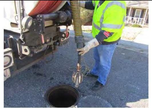
11. If the sewer hose will run over the edge of the manhole frame, or if the manhole is off-road, use an upper manhole roller to protect the sewer hose while cleaning the pipe.
