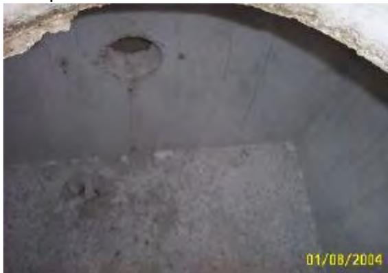
Single hole in baffle wall
