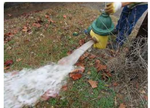
2. Attach the water fill hose to the hydrant, making sure the hose will not kink during filling.
