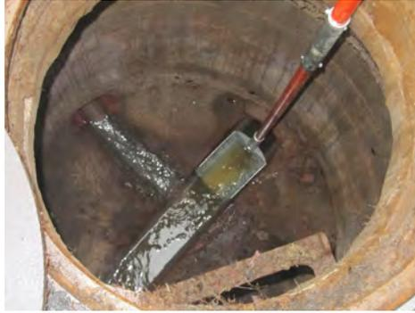
**Photo 7-3. Debris Trap Placed in Manhole Channel**
