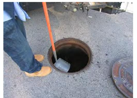
14. Activate the nozzle with low water pressure to verify visually that the nozzle is working properly, and then gently increase water pressure.
