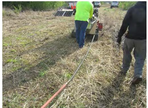
2. Use axes, machetes, or Gerber knives when necessary to expose hazards and obstacles such as elevated manholes, force main cleanouts, and cables that could be damaged by the easement machine, cause injuries, or become entangled in the equipment.
