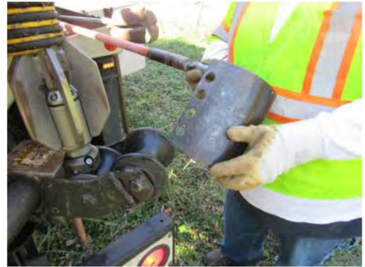
13. Lower the trap into the manhole, and position the trap to catch materials at the downstream pipe invert.
