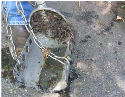
**Photo 7-6. Examining a Debris Trap for Signs of Light Roots**
