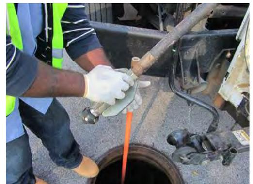
10. Lower the nozzle and tiger tail into the manhole channel.
