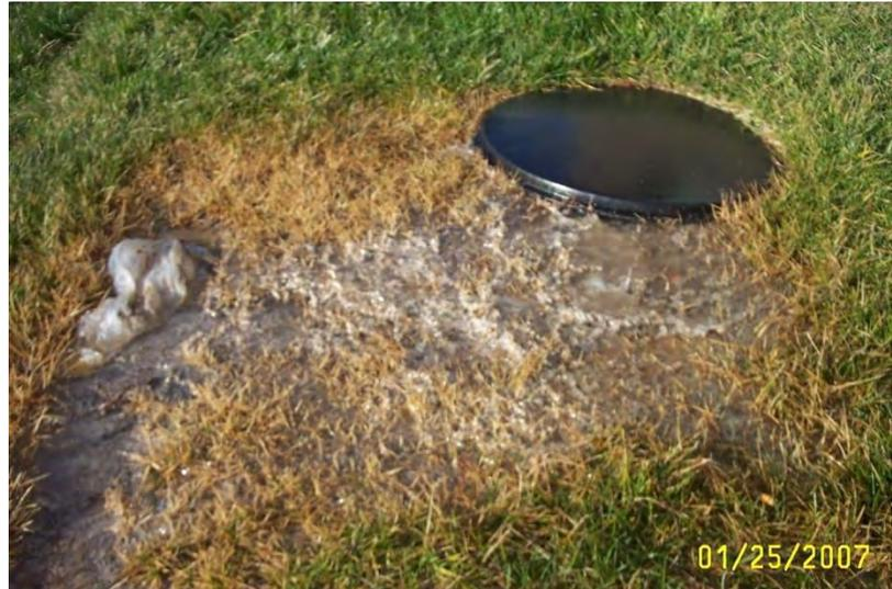
Grease Traps that are overflowing. This needs to be reported to the Health Department and Stormwater personnel. The FSE manager/owner needs to be immediately notified that the grease trap should be pumped as soon as possible.
