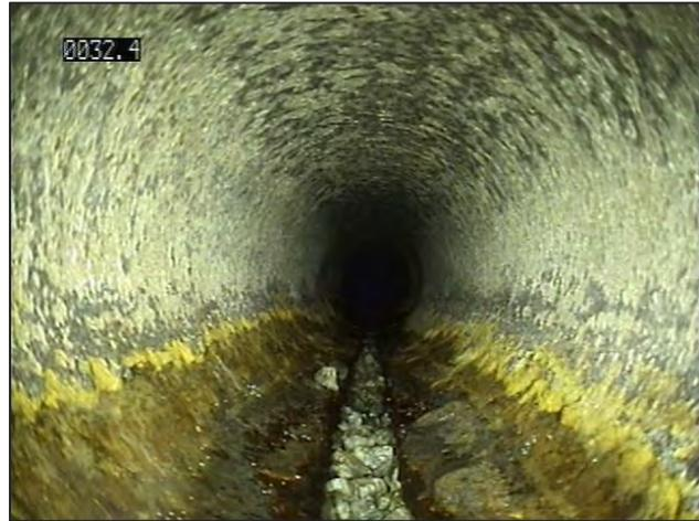
**Figure 3. Ductile Iron Pipe Invert Corrosion from Acidic Discharge**
