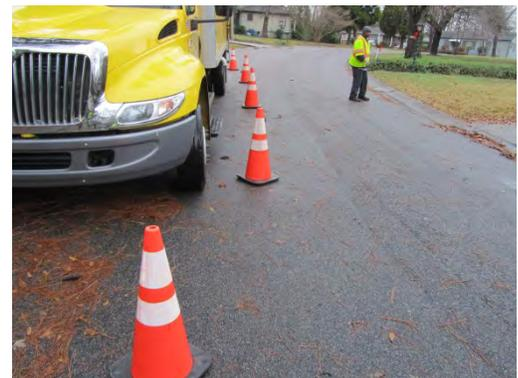
For off-road pipe inspections, position the TVI van in the best location to accommodate the camera cable as it is pulled off the reel to the remote manhole.
