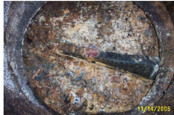
Floating flexible plastic "U shaped" outlet T that has become dislodged from the trap wall.
