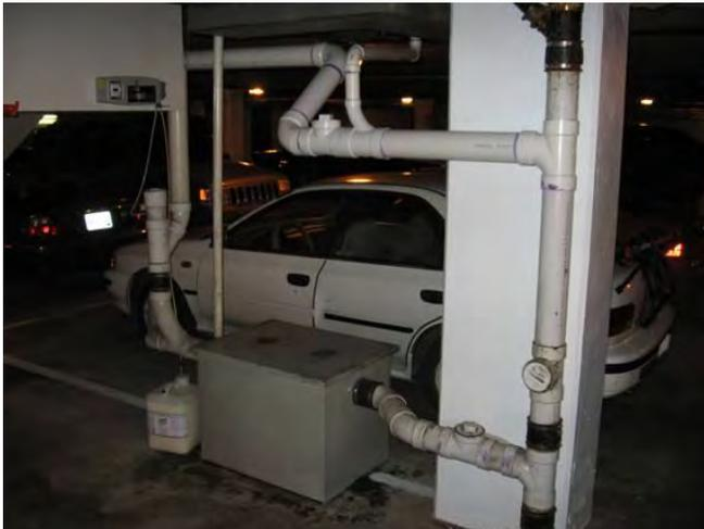
**Additives**, with automated feed system, connected to the front of the Grease Interceptor (this one is located in parking garage below a FSE). Additives (acids, caustics, soaps, surfactants, enzymes, etc...) should never be allowed prior to a grease interceptor!
