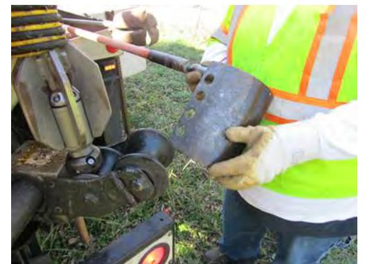
13. Lower the trap into the manhole and position the trap to catch materials at the downstream pipe invert.
