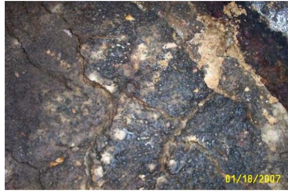
No outlet T located due to depth of FOG, no Grease trap maintenance! Noncompliance
