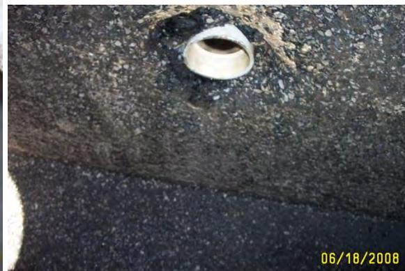
Outlet chamber side view of PVC sweep (90 degree portion
