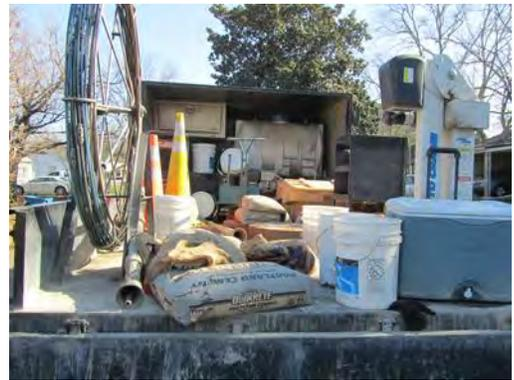
1. Upon arrival at the site, position the Crew Truck in the best manner that provides direct access to the manhole and limits exposure to traffic.
