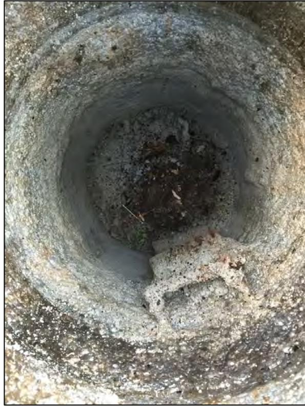
Figure 1. Concrete Manhole Corrosion from H<sub>2</sub>S Gas
