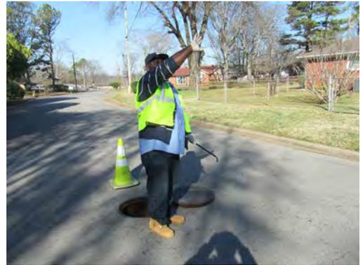
17. A proofing tool can be used to determine if there is material remaining in the pipe after cleaning.
