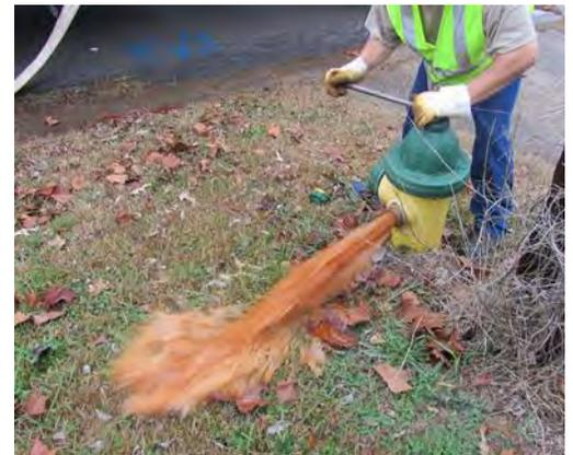
After the water runs clear, slowly close the hydrant valve to avoid water hammer.
