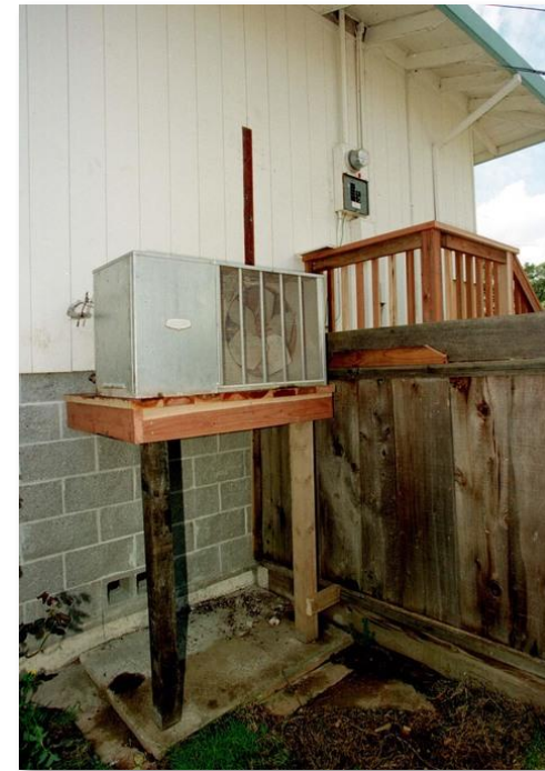
FEMA Hazard Mitigation project in Alabama - Raising this utility box prevents future damage in the event of a flood. Photo by: Dave Gately/ FEMA News Photo
