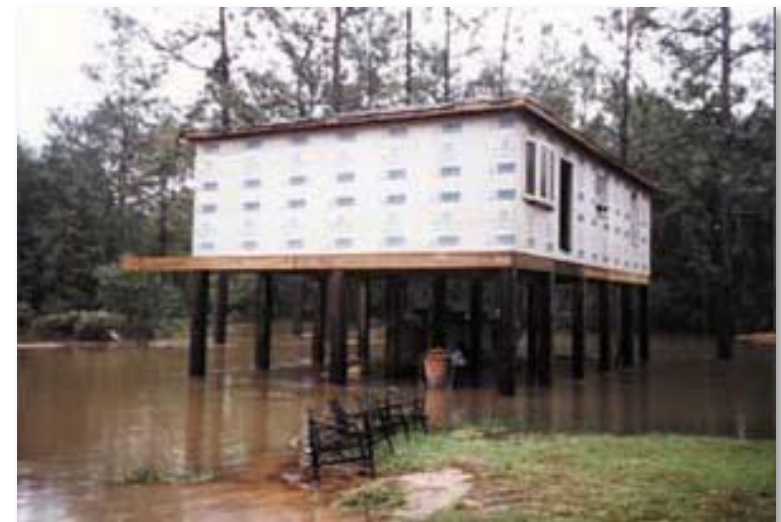
Baldwin County, Alabama – Residential elevation and installation of breakaway walls saved this home from flood damage. FEMA News Photo
